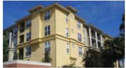
Multifamily Residential Building, 141 Chestnut St.
